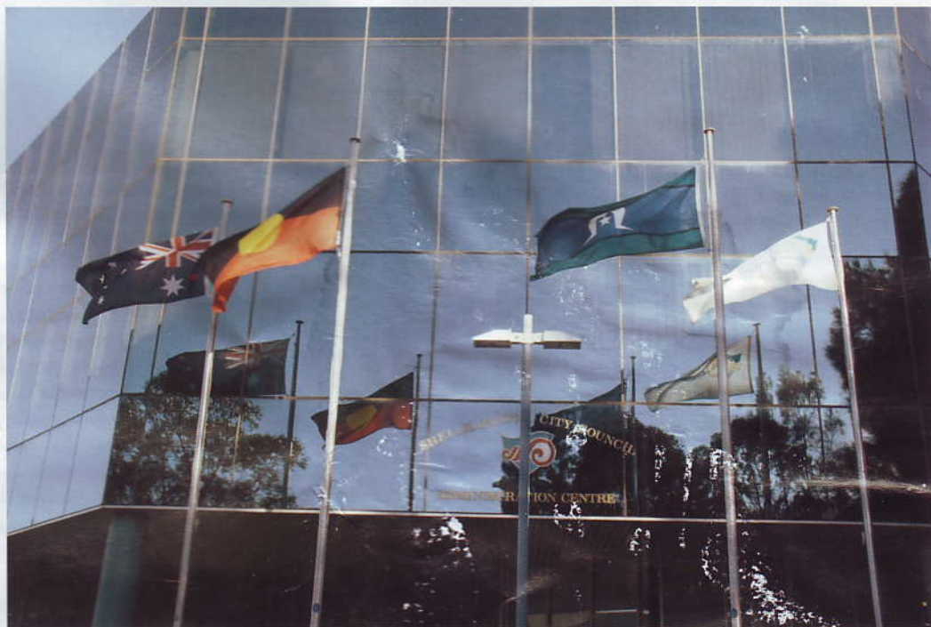
Lamerton House in Shellharbour ... 30 per cent energy saving by installing T5s
